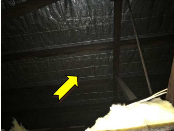
Photo 7. Interior, throughout, underside of roof – suspected SMF sarking insulation material.
