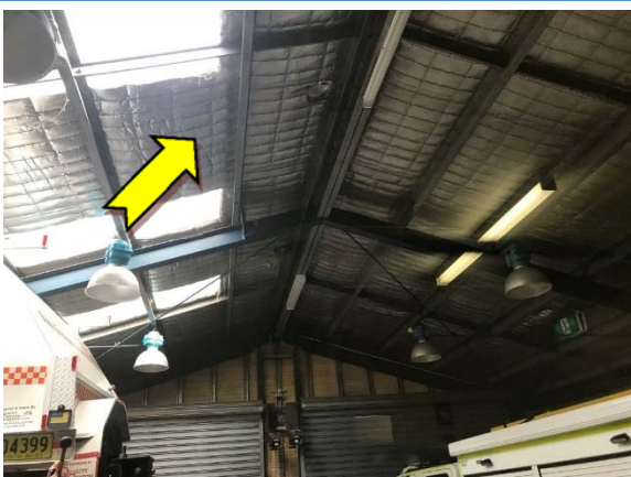
Photo 5. Exterior, garage, underside of roof – suspected SMF sarking insulation material.
